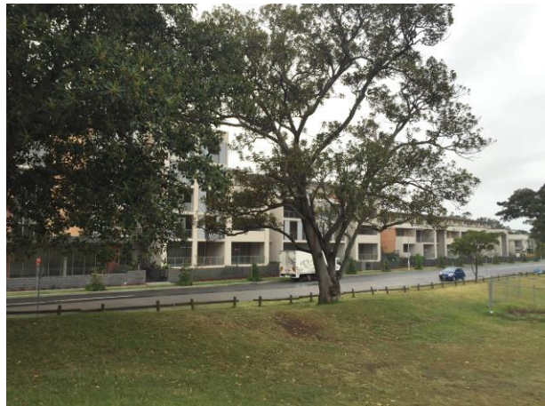
PICTURE 2.8 – NEW APARTMENTS, JASMINE STREET
