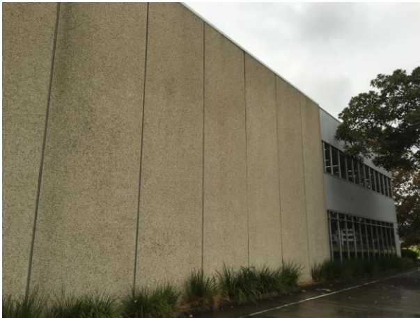
PICTURE 2.3 – TYPICAL BUILDING CONSTRUCTION
