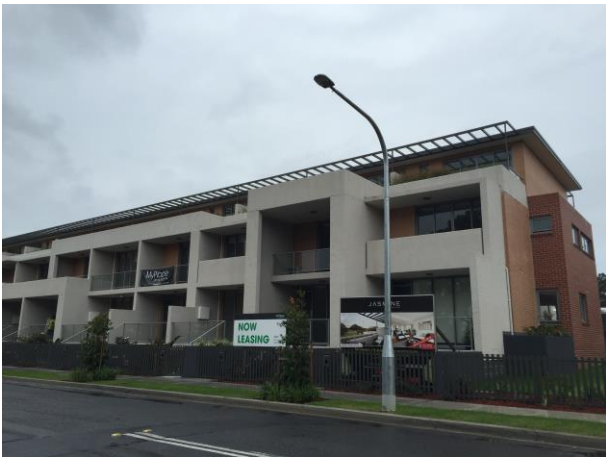
PICTURE 2.7 – NEW APARTMENTS, JASMINE STREET
